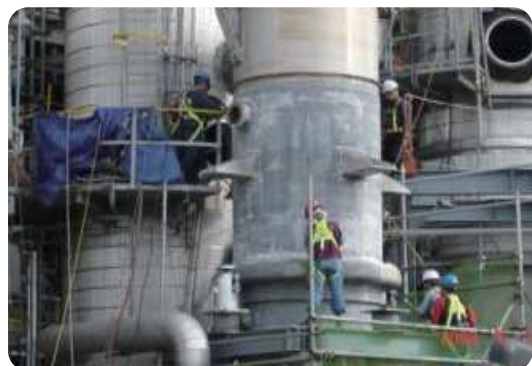
| REVAMPING PROJECT REACTOR 설치 |
