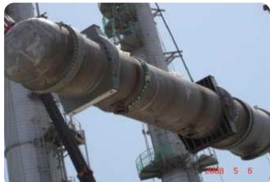
| REVAMPING PROJECT REACTOR 설치 |
